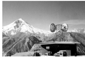
Construction of satellite telecommunications system in Iran
