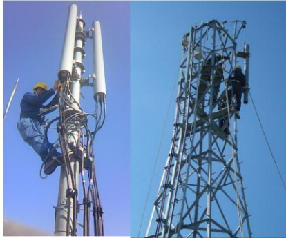
Construction of base stations for mobile phones
