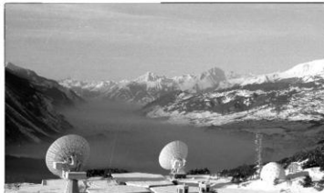
Construction of satellite telecom system in Switzerland
