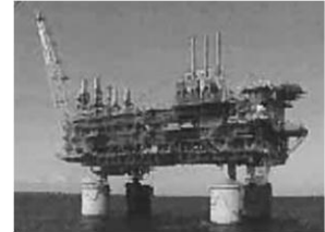
Construction of network for an offshore oil field plant
