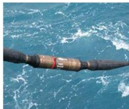
Submarine cables and Submarine seismometer system
