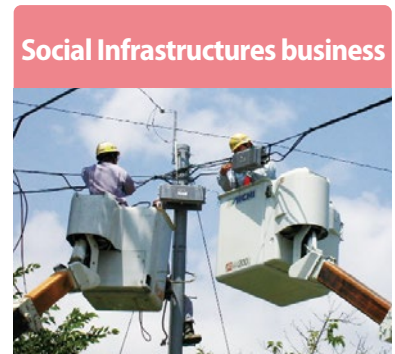
CATV System Construction
