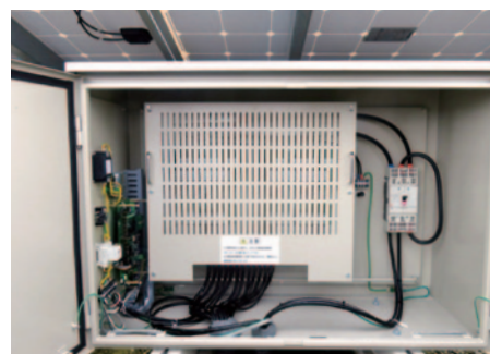
Junction box with a remote monitoring device
