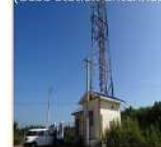
(Base station antennas)
