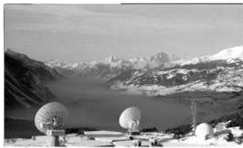
Construction of satellite telecom system in Switzerland
