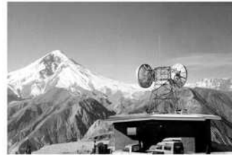
Construction of satellite telecommunications system in Iran
