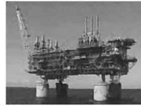
Construction of network for an offshore oil field plant
