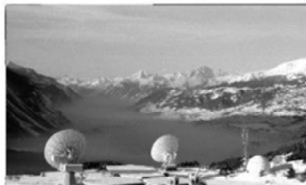
Construction of satellite telecom system in Switzerland
