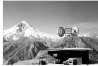
Construction of satellite telecommunications system in Iran
