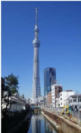
Installation of digital terrestrial broadcasting equipment on Tokyo Skytree
